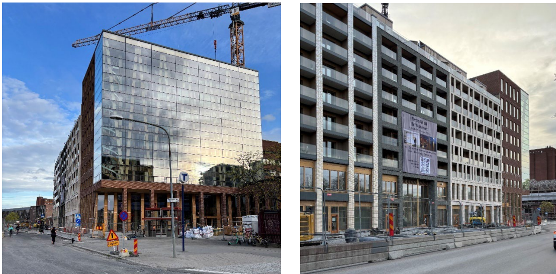
Figure 1. Electrolux new HQ in Kungsholmen, left: from the front, right: from the back with the connected residential building, Brf Gourmet.
